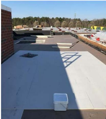
The roofing portion of this project consisted of more than 30 individual roof areas, some to be torn off and others to be retrofitted. The basis of design was a 30-year Sarnafil 080 S-327 MEMBRANE installed as a Rhinobond system on the nailable substrates (metal decks) and Adhered assemblies on the non-nailable (structural concrete) roof areas. The insulation requirements varied dependent upon the exiting roof assembly R=Value to achieve a finished R=Value of 30.
